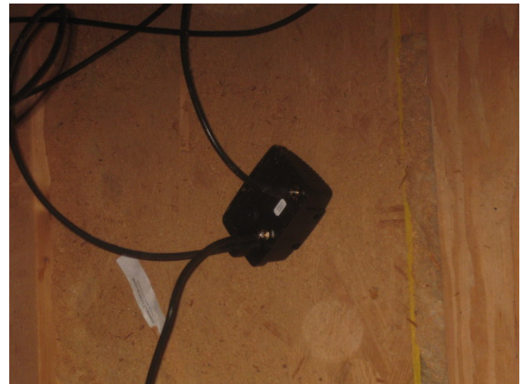
AntennaCraft 10G222: 29 DB each in VHF and UHF with separate Coax Inputs and Internal Combiner to Single Coax Output
