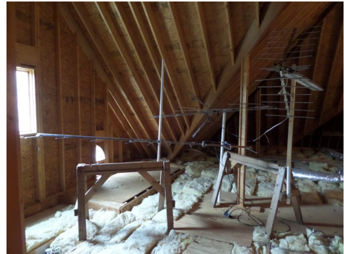
Bottom = VHF Yagi Aimed at Savannah; Right = Channel 16 UHF Deep Fringe Antenna Aimed at Whitehall SC
